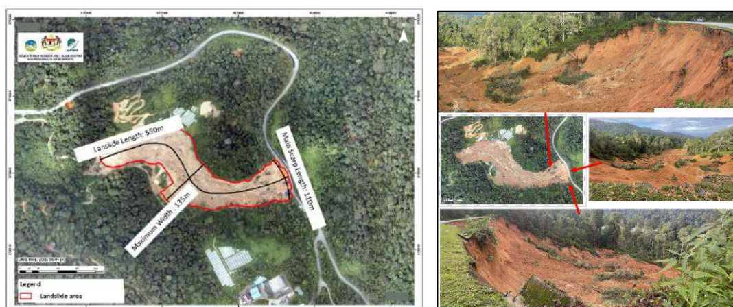
Fig. 3: Dimension of the landslide and the photo of the main landslide body.
