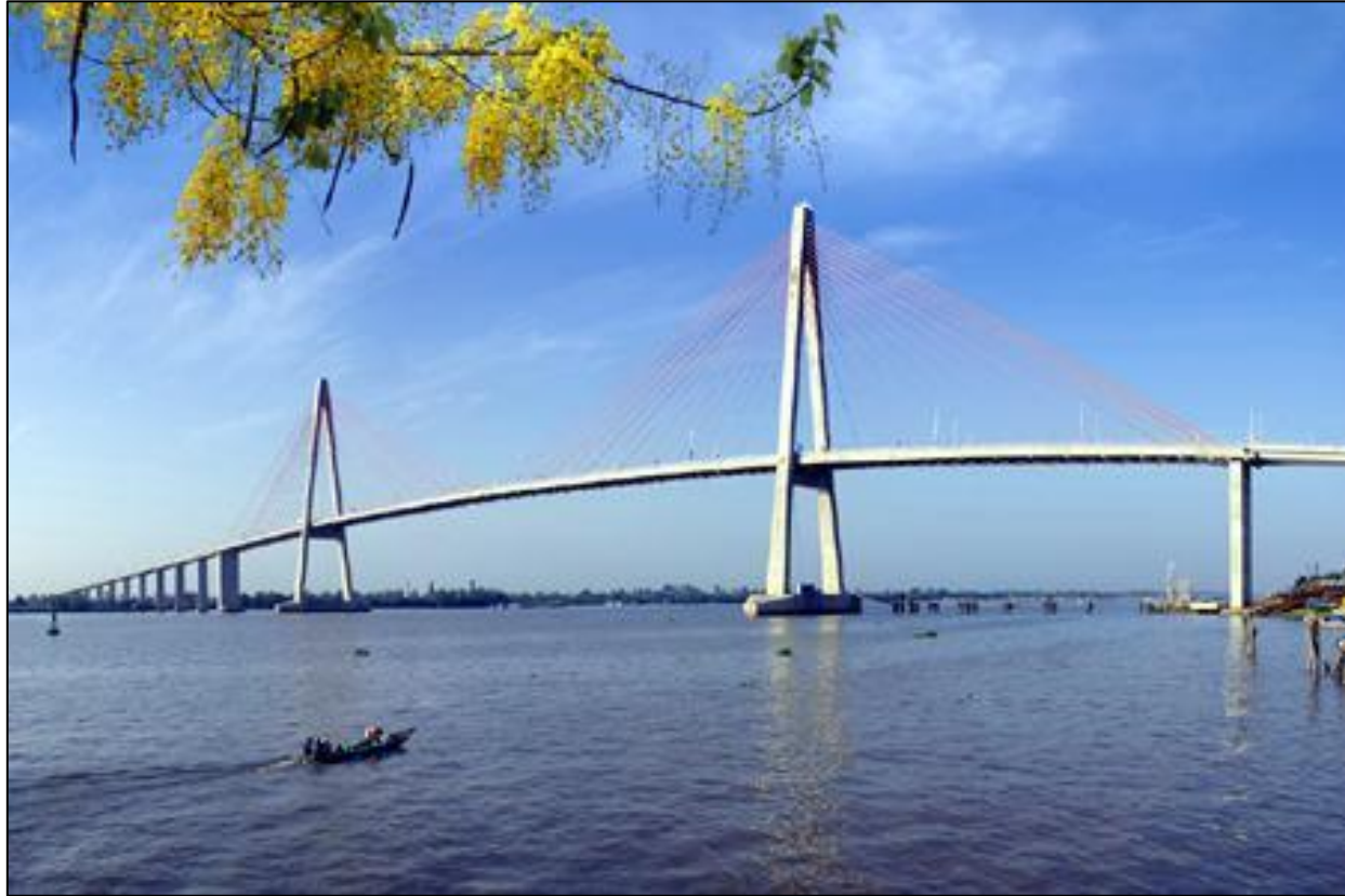
Figure 4.10 Rach Mieu Bridge.
