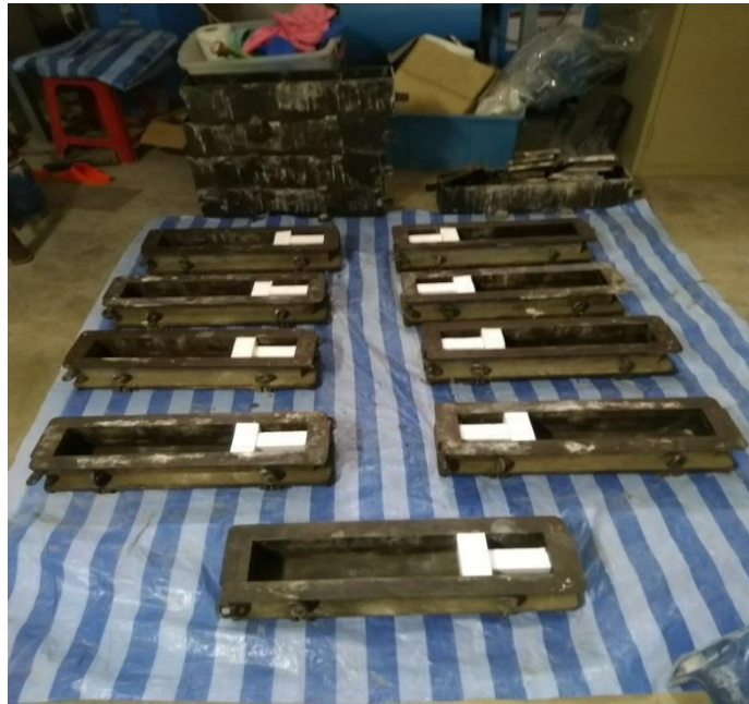
Figure 9.5 Preparation for concrete beam casting in the steel molds
