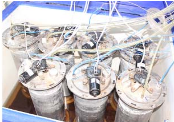
Fig. 3.37 Seven digestion tanks with gas tube
