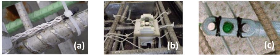
Figure 1. Installation example of Ag electrode and two MEPs (ECI-2 and CPMP-2).
