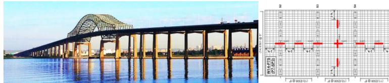
Figure 2. Newark Bay Bridge and typical sensor layout in the precast deck panels.
