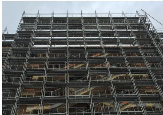
Figure 2. Modern scaffolds used in construction sites.
