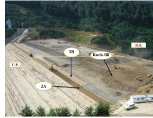
Figure 6. The dam body cross-section.
