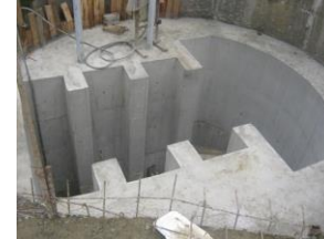
Figure 10. Vertical shaft of intake structures.
