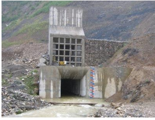
Figure 5. The diversion tunnel.
