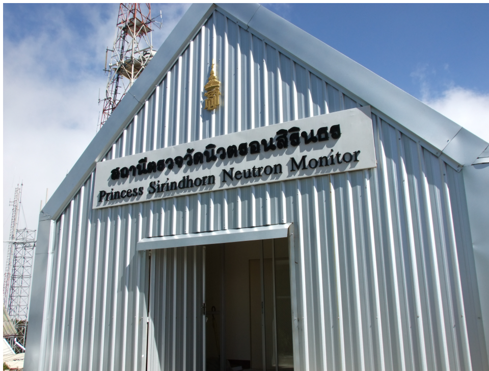
Figure 3.2: The building of the PSNM station.
