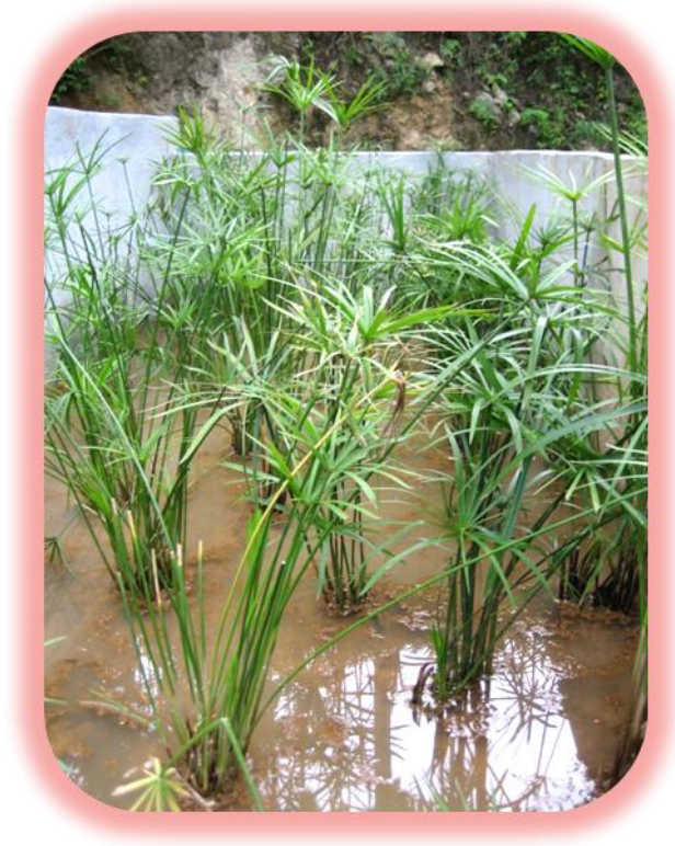
Figure 4.3 Constructed wetland pond with Cyperus spp.
