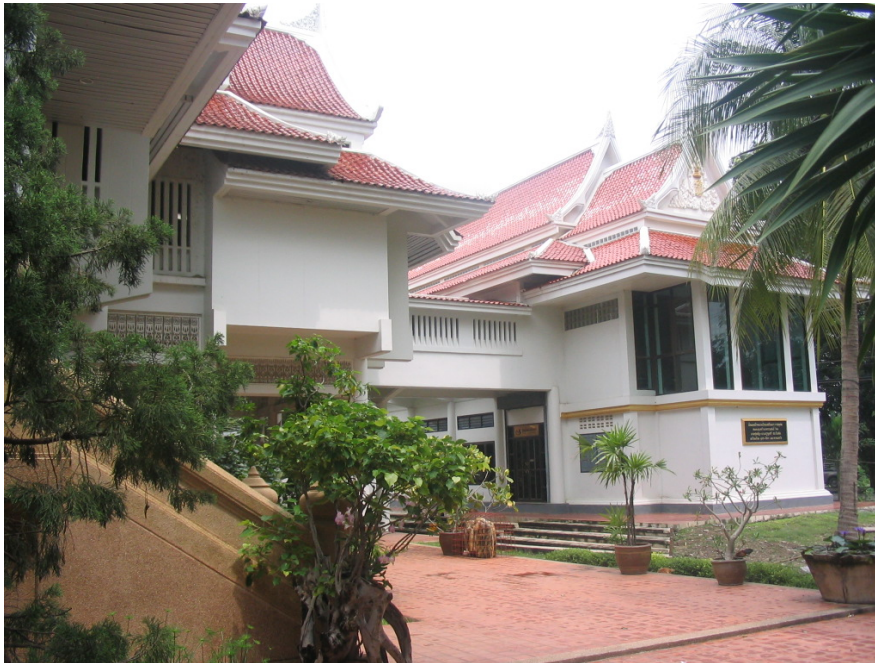
Figure 14 Presents the bridge that connects the main building to the sub-building that shows the architectural: character of the Muang Temple Folklore Museum.
